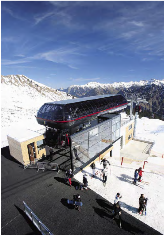
Kronplats Gondola System Top Station
